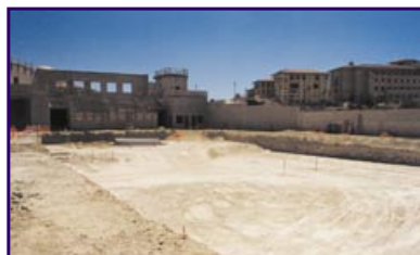
Excavation of the university's Olympic-sized swimming pool has begun.
