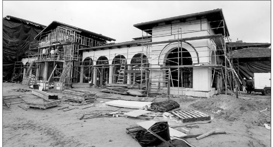
Construction on the SUA, Aliso Viejo campus is progressing steadily.
