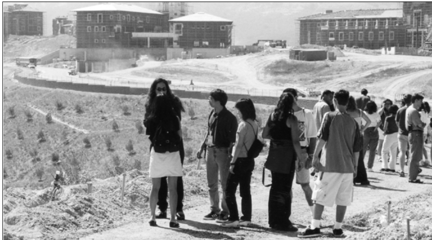
A tour of the Soka University of America, Aliso Viejo, campus under construction.
