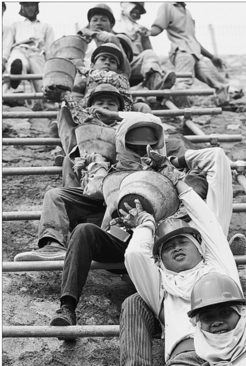
Workmen in Indonesia.
