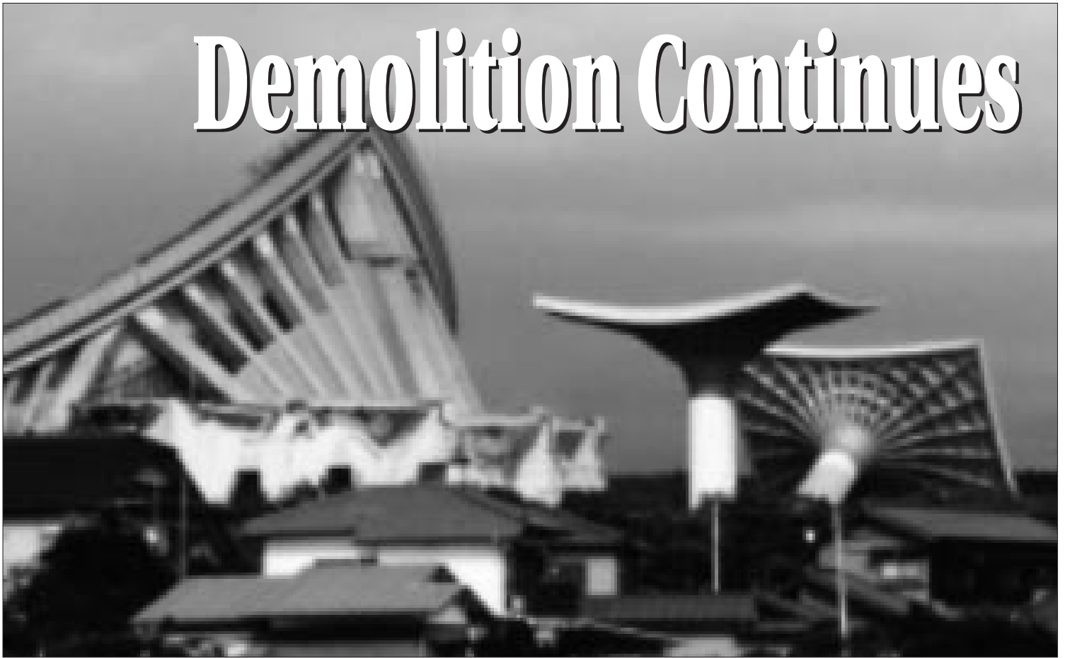
Above, a column falls in the one-time Pavilion of Perfect Harmony at the entrance of the Grand Main Temple. Five columns of polished marble from Greece with inset pre-cast concrete panels used to tower above burner-finished granite paving that was inlaid with polished marble mosaic patterns. Below, the Mystic Sanctuary, patterned on a crane about to take flight, now stands stripped and empty. At one time, it was composed of a dynamic and richly curved roof. Photos courtesy of 'Kaikaku Jiho.'
