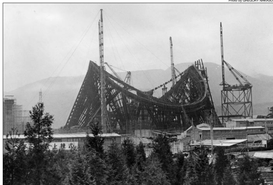
About 120 engineers worked on the Grand Main Temple project, determined that the building would stand for hundreds of years. Some 23,500 tons of steel — the type used in shipbuilding — were used in the framework.
