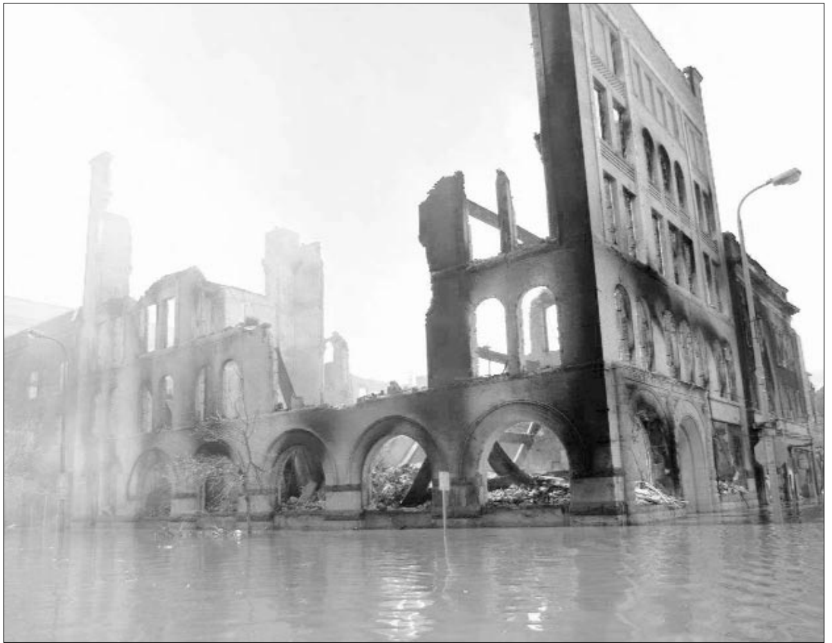
The Security Building in Grand Forks, N.D., smolders on Sunday, April 20. Fires broke out after the floods and at least six buildings were destroyed.
