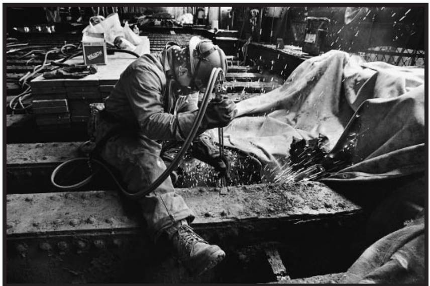
Welder, Manhattan Bridge.
